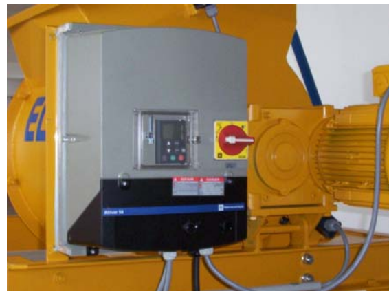
Frequency-controlled mixer shaft rotation.
